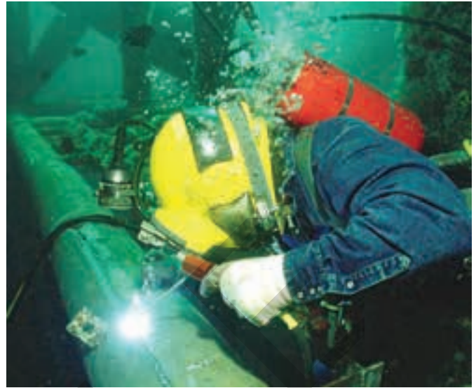
Figure 25-2. A welder making a fillet weld on a pipe reinforcement, or doubler. Wet welding is a Class B weld per AWS D3.6M code.
