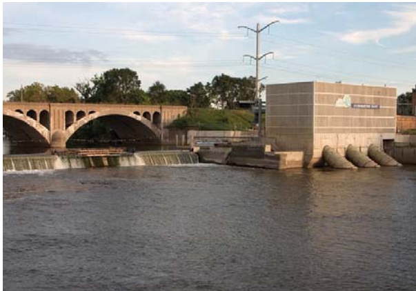
Figure 5-11. Hydroelectric power can be even generated by small rivers and low dams. This plant, operated by a small midwestern city, generates enough electricity to operate a sewage treatment facility serving several adjoining communities.
